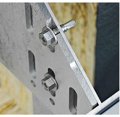
**Sliding point.** When the aluminium framework is fixed to the cladding support, it is imperative that the self-drilling fastener SDA5 be inserted in the middle of the slotted hole with overtorque to ensure a tension-free installation.
