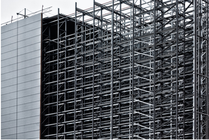
High rack construction
